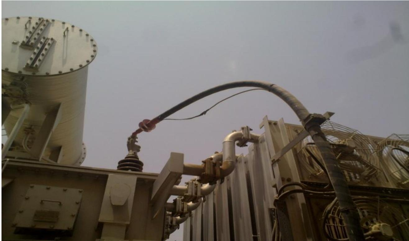
For the purpose of stealing the bus-bar and neutral cable vandals connect the neutral cable with the earth cable. By that act personal and asset will be in major danger of transformer fire and explosion
