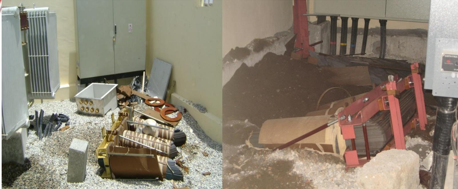
These transformers contain windings which are made of pure copper and consider as the most target for theft due to the high price of stolen copper
