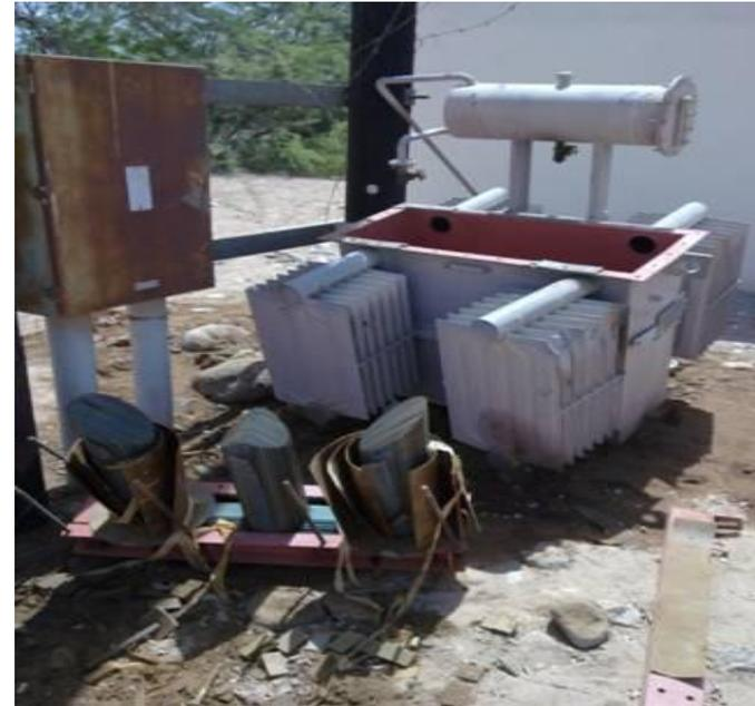
The main target in such transformer is the winding which also made of pure copper. Vandal's shutdown the transformer by pulling the Dropout Fuse (DO FUSE) After that, they drop the transformer to the ground and stealing the copper.
